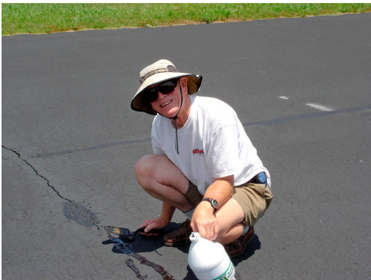
Bill Dodge hard at work on your runway, filling those pesky cracks that grow wider and deeper every year.
